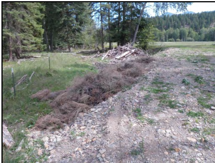
Figure 7. Photograph of weed disposal area. Fill removed from the floodplain in the Demonstration Phase was used to expand the road grade and bury weeds.
