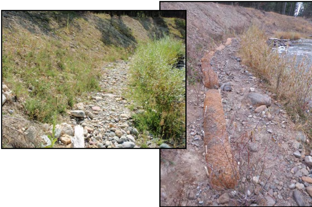
Figure 3. Photographs of revegetation of the terrace slope using 16-inch high density coir logs, 16-gallon willows, and one and two-gallon shrubs. This treatment was focused on the interface of the terrace slope and bankfull bench. Photograph on the left shows the bench prior to treatment. Photograph on the right shows the bench after treatment.
