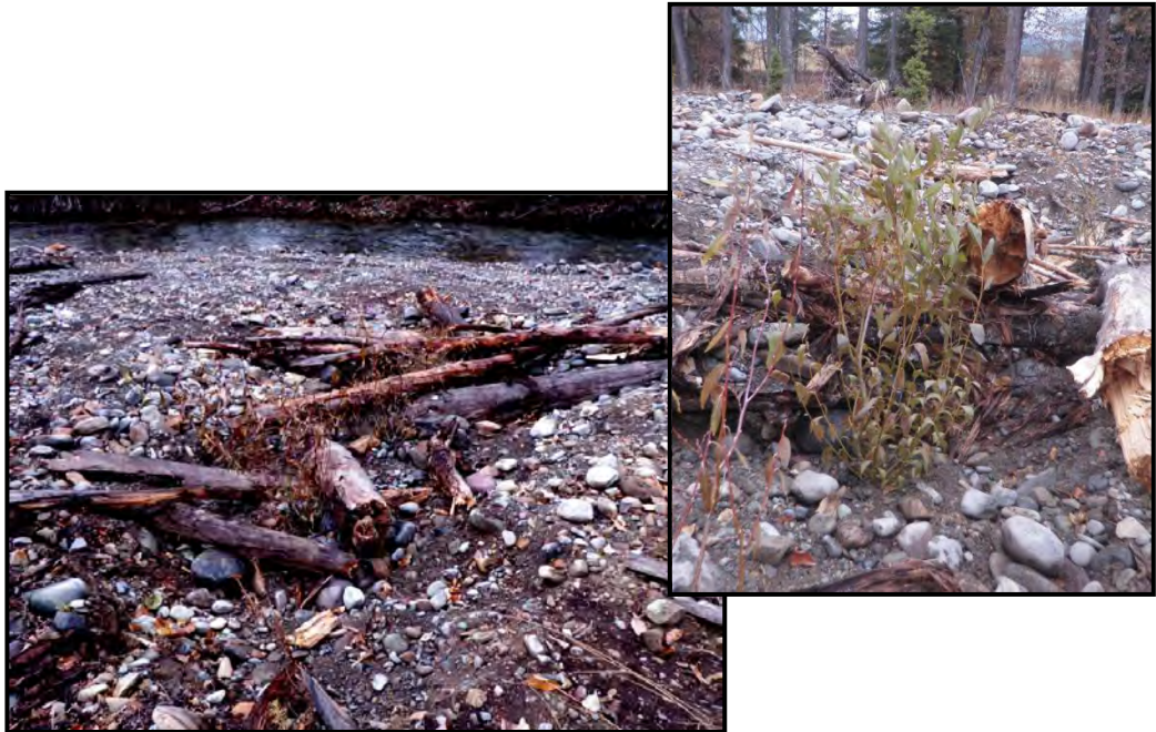
Figure 5. Photographs of a constructed floodplain swale planted with 16 gallon Drummond willow. Large woody debris was partially buried into the floodplain during swale construction, and coarse woody debris was placed around planted shrubs to create microsites.
