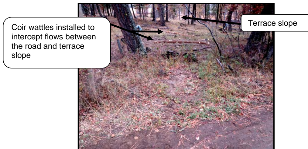
Figure 9. Photograph showing the concentrated route of road run-off leading to the top of the terrace slope in the Demonstration Phase. Coir wattles were installed in a staggered pattern to reduce the velocity of overland flows, shorten the effective slope length, and prevent further erosion of the slope.
