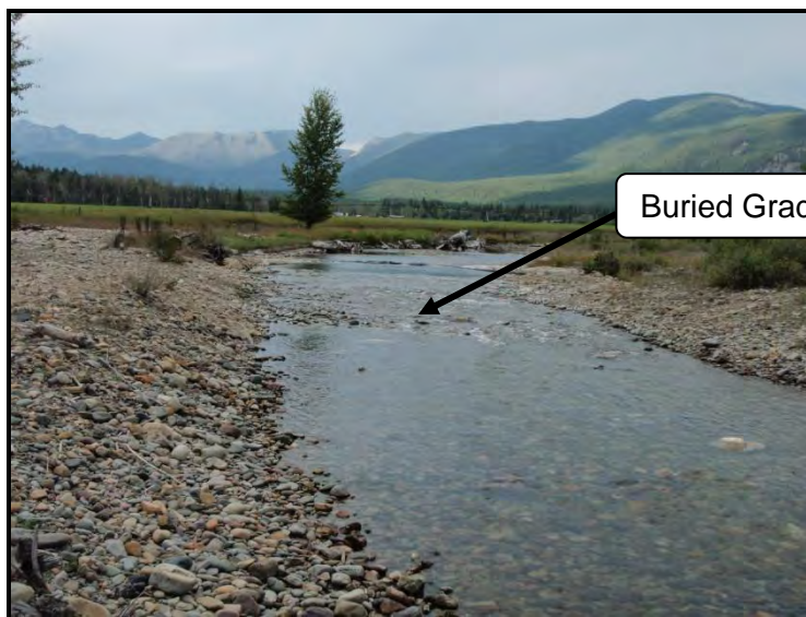
Figure 8. Photographs of vane maintenance in Phase 2. Top photograph shows the structure prior to installation of the boulder grade control. Photograph on the bottom shows the structure after installation of the boulder grade control which reduced the drop over the structure from 2 feet to approximately 0.5 feet.
