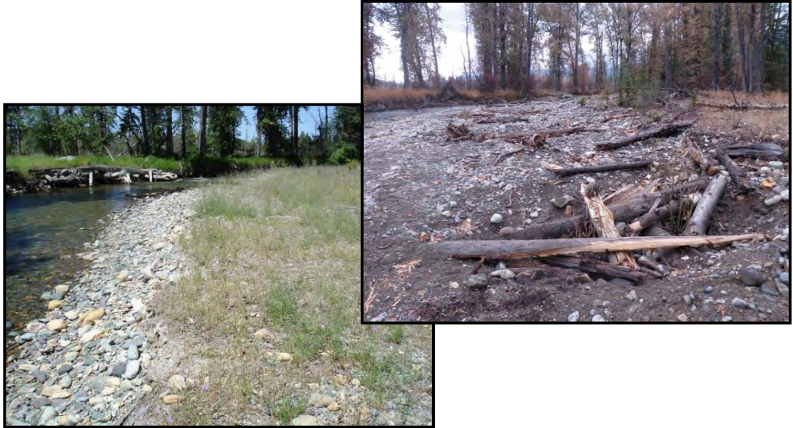
Figure 4. Photographs of Demonstration Phase floodplain surface before (left photograph) and after (right photograph) removal of 400 cubic yards of material, construction of floodplain swales, and placement of woody debris and 16-gallon willows in swales.
